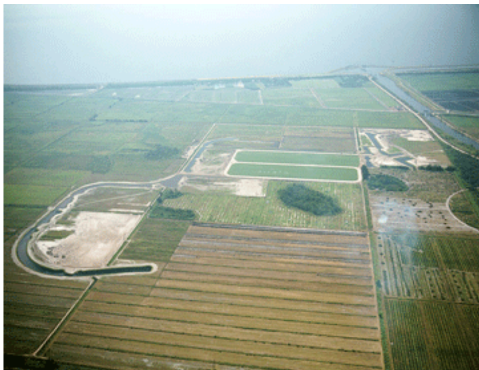
Aerial view of the Lake Point Project showing the proximity to Lake Okeechobee to the West. The Lake Point land is more than 20 feet high to the elevation of the Lake that goes between 11 and 14 feet.
